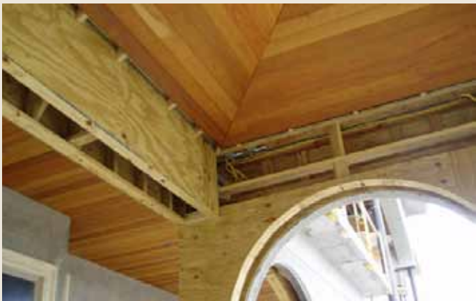
Cavity wired for installation
