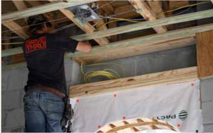
Cavity over arch being wired for 110V AC
