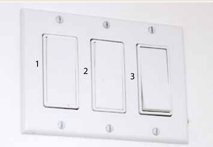
Individual switches can be wired to control power to each unit independently; multiple switch panels can also be used
