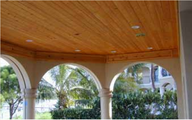
Recessed screens mounted within multiple arched openings, with removable front access panels
